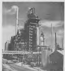
A MAJOR customer of the powerhouses is Lago's Cat Cracker which uses electricity, steam, water and air. UN CLIENTE grandi di powerhouses ta Cat Cracker di Lago cual ta usa coriente, stien, awa y aire.
